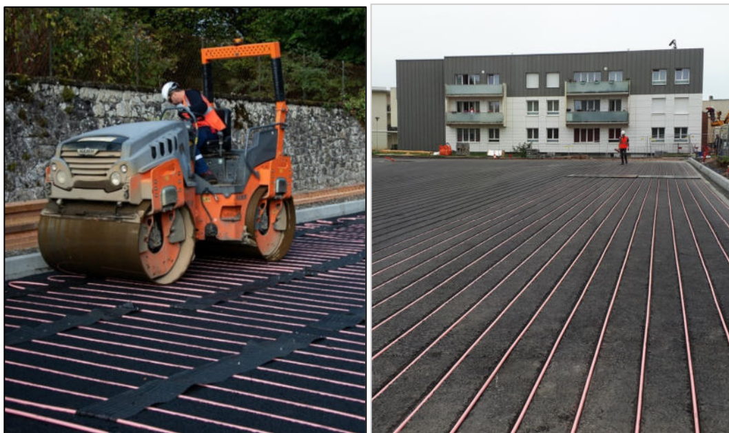
Fig. 1: Power Road pipe installation - (left) Indentation installation method - (right) Grooving installation method
