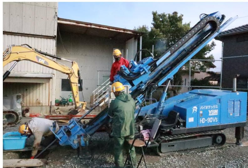
Fig.2 Drilling equipment in Japan
