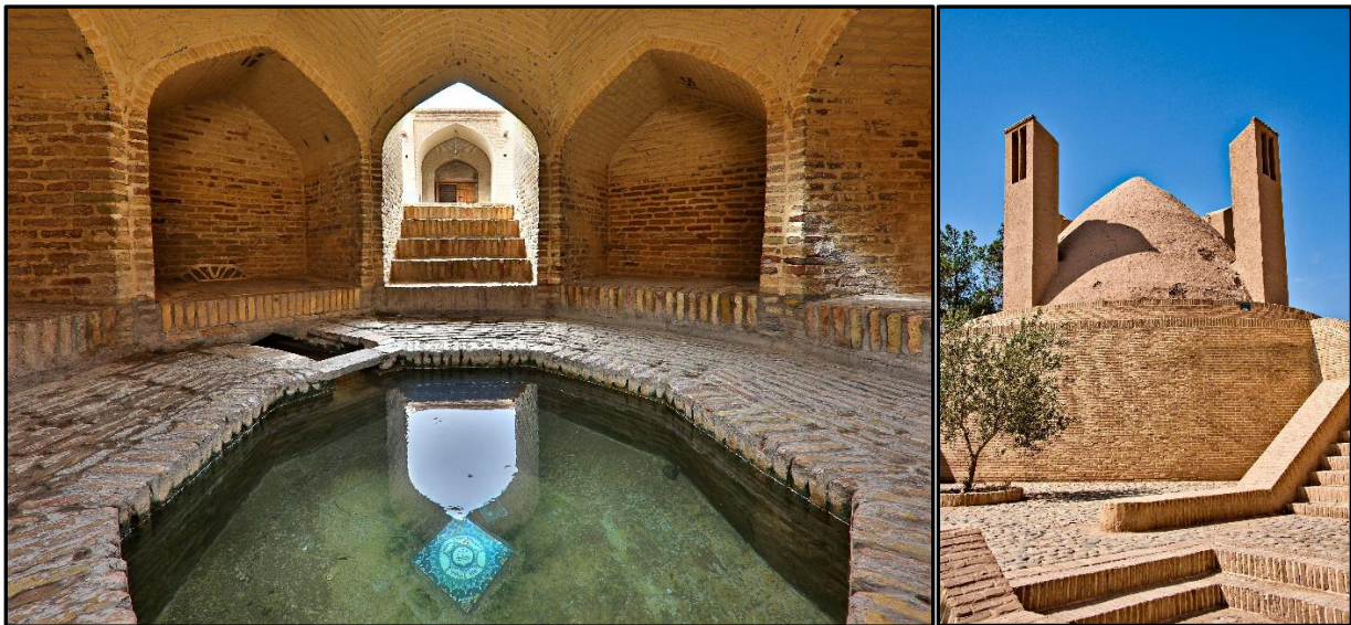
Figure 8 (Left): Inside of the Klar Ab-Anbar in the Shah Abbasi Caravanserai, Meybod, Iran (MehmetO 2018)
