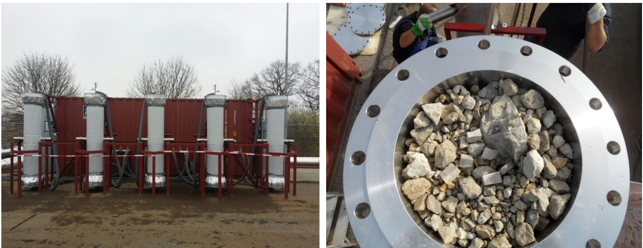
Fig. 3: (a) Bypass system in Kirschweidach and (b) Reaction columns while being set up
